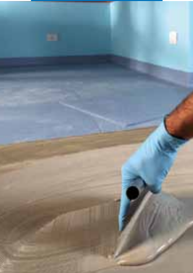
Applying Ultrabond Eco 380
