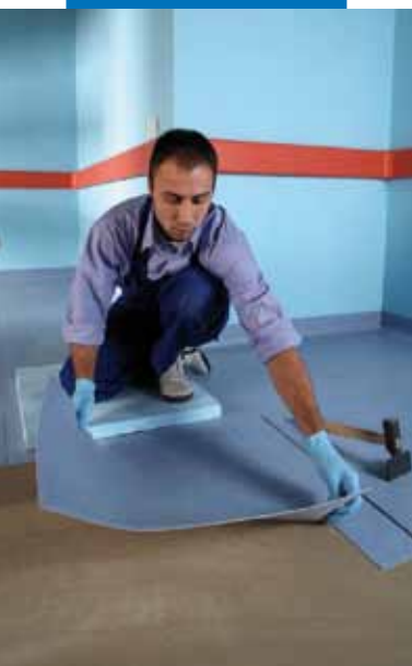
Installing PVC floor tiles
