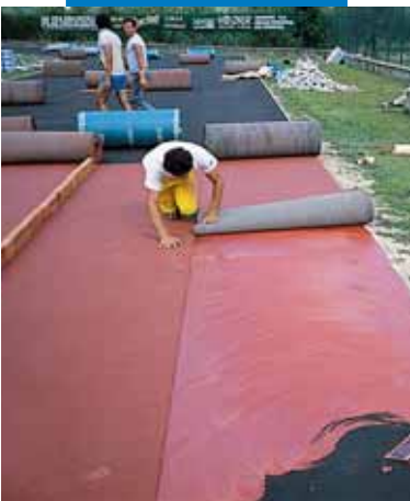
Installing rubber flooring with Adesilex G19
