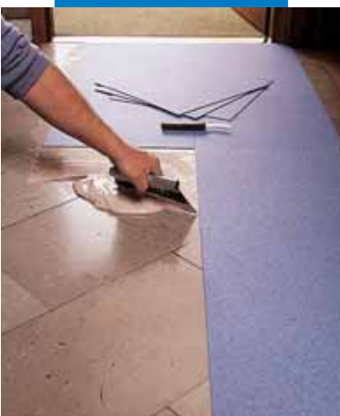
Laying PVC on a non absorbent substrate with Adesilex G19
