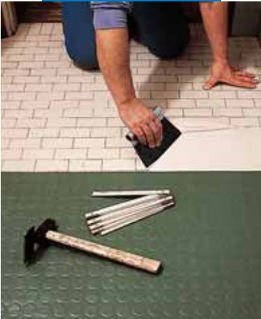
Spreading Adesilex G19 with a notched trowel
