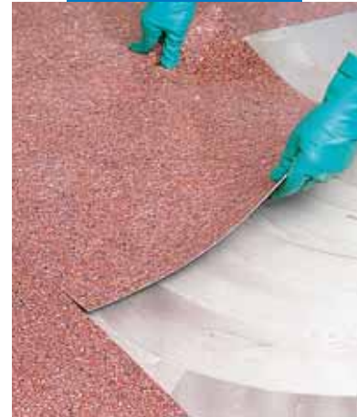
Installing PVC with Adesilex G19
