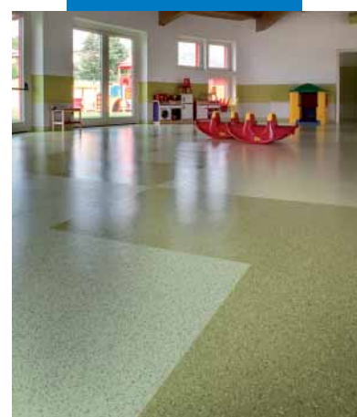
An example of installing rubber flooring in a school: Municipal Infants School, Carobbio degli Angeli (Bergamo)
