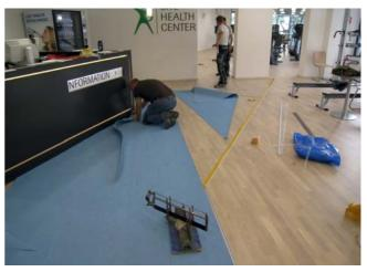
This is a typical situation easy to master with UZIN KE 2000 S NEW: Installation of PVC floor covering during ongoing operation on an installation underlay, here, for example, on UZIN RR 186.
