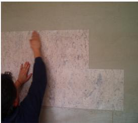
Align one corner of the tile against the two axes and then carefully place down the rest of the tile.
