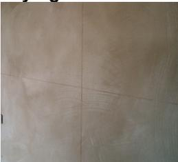
Find the centre of the wall using a chalk line, draw two symmetrical axes and use these as a starting point.
